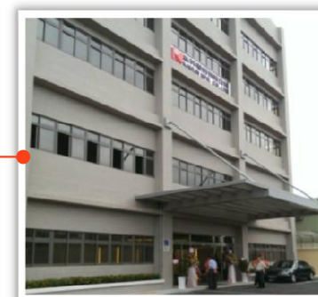
Taoyuan (16,500 M 2 ) Assembling Capacity : 120K Unit/Y
