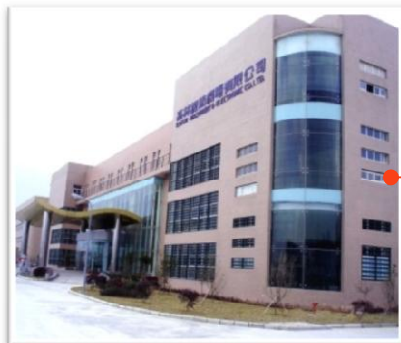
Ningbo (95,461 M 2 ) Capacity : 360K Unit/Y
